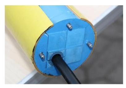
Install RM pass-through and RM solid compensation modules in the pass-through frame.
