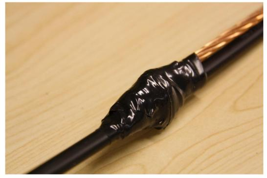
Protect the joint with the vulcanized tape that comes with the joint closure.
