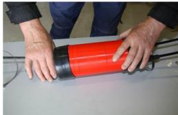
Push the end pieces over the frame tube all the way to the end.
