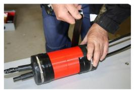
The tape is installed by stretching it into place.
