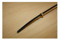
The hose clamp has been installed loosely to one of the FTTH cables.
