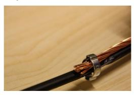
Position the hose clamp in a way that makes sure sufficient connection is made. Flatten the end of the grounding wire and place it between the cable and the hose clamp.
