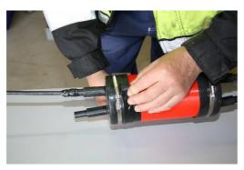
When the beginning of the tape sticks, turn the tape around the case while slightly stretching and pressing it into place.
