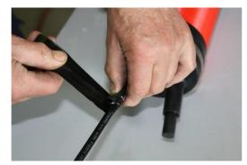
Seal the cable glands with vulcanized tape that comes with the joint closure. A piece of tape about 15 cm long is sufficient to seal the cable glands. When the end of the tape sticks, stretch the tape and turn it over the cable gland, pressing it tightly against the exit point of the cable.
