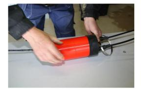
Pull the frame tube on the splice tray along with the rubber cable glands.
