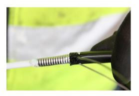
Heat the sheath, starting from the point where the cable is peeled, at a length of about 10 cm, and remove the halves of the sheathing from the corrugated steel plate. Cut off the steel sheath and the reinforcements under it 3–5 cm from the starting point of peeling. Pull the sheath out from the end of the cable.
