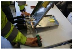
You can lock the upper splice tray in an upright position by tightening the screws.
