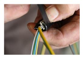
Protect the connector of the grounding wire with insulation tape. After that squeeze the sheath halves against each other and tape them together.
