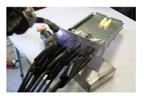
Heat the shrinks into place, starting the heating from the flange of the joint closure.
