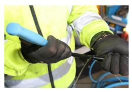
Another method of peeling is to split the sheathing with a knife from the grooves of the steel wires at a length of about 20 cm.
