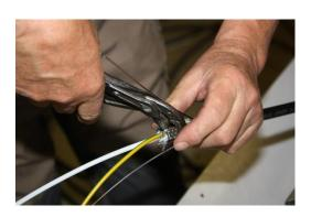
Scrape off the white ribbon under the armoring from one of the sheath halves and the plastic layer on the surface of the armoring. Flatten the end of the cable sheath with pliers and squeeze the connector of the grounding wire onto that half of the sheath.
