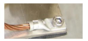
Attach the grounding connector under one of the screws in the case.
