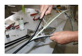
Bend the cable slightly to separate the halves of the cable at the peeling point. Pull the cable halves apart while taking care not to damage the fiber tubes. Cut off the halves of the sheath so that the remaining pieces are about 3 cm long. Cut off the reinforcements under the sheathing.
