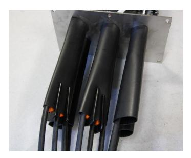
Thread the shrinks over the cables and guide the ends of the cables inside the closure.
