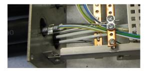
The corrugated steel sheath of the FZVD2PMU Flex cable is connected to the grounding rail with the help of an Oetiker hose clamp. It connects the steel sheath and the wires. The Wires are then connected to the grounding rail.
