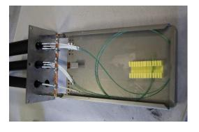
Lay out the fibers on the splice tray and cut off their excess lengths.
