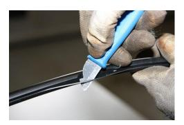
Dig out the steel wires. Cut the steel wires at a length of about 10 to 15 cm.
