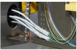
To save space, it is a good idea to attach the fiber tubes of FTTH cables in bundles to the splice tray, but at most 4 tubes per bundle.
