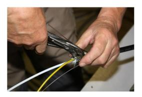
Use a knife to scrape off the white ribbon under the armoring from one of the halves of the cable sheath. Also scrape off the plastic layer on the surface of the armoring. Carefully install the grounding wire.
