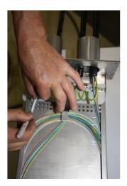
Mark the starting points of peeling on the fiber tubes, cut the fiber tubes without damaging the fibers, remove the gel on top of the fibers and attach the fiber tubes to the splice tray.
