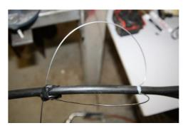
Bend the steel wires backwards and lock them with e.g. insulation tape to prevent damage from their sharp ends.
