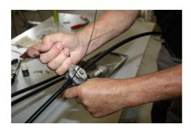
Split cable sheath using ST-OCS splitting tool. Guide the tool blade into the groove of the steel wire and pull the sheath open on both sides of the cable.
