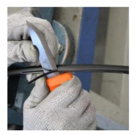
Peel out the steel wires or fiberglass strength members of the cables along the entire length to be peeled.
