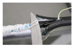
Push the binding threads of the fiber tubes towards the cable to loosen them, and cut them at the base of the sheath.
