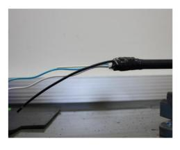
Protect the connector of the grounding wire with insulation tape. After that squeeze the sheath halves against each other and tape them together
