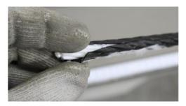
Open up the middle sheath from the end with a knife, enough to get a gpip from the edges.
