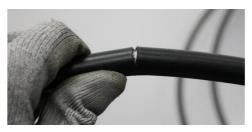
Bend the cable in different directions at the incision point to break the steel band.
