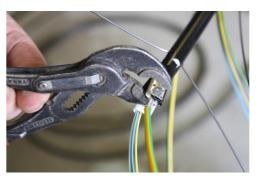
Flatten the end of the cable sheath with pliers and squeeze the connector of the grounding wire onto that half of the sheath.
