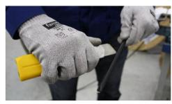
Split the sheath from the end of the cable from the grooves of the strength members for about 15 cm.
