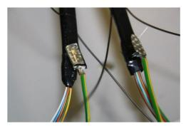
The connectors of grounding wires installed into FZVD2PMU Flex direct buried cables. Notice the protection of fiber tubes against one of the halves of the cable sheath.
