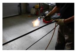
Clean the cable from any dirt and heat the cable sheath over the entire length to be peeled. This makes peeling easier, as the cable sheath material is HDPE, which is harder material than the LDPE traditionally used in outdoor cables.
