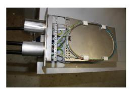
The uncut fiber tubes are attached to the underside of the splice tray with the adhesive fasteners that come with the joint closure.
