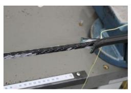
Cut the halves of the sheaths to about 3 cm in length and remove the white swelling strip and its binding threads from the middle sheath. Also cut the tear wires at the base of their splitting grooves.
