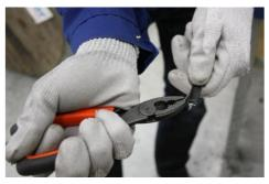
Bend out the ends of the steel wires or fiberglass strength members and pull them out of the sheath along the entire length to be peeled.
