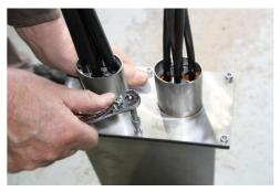
If you are using a battery-powered screwdriver to tighten the screws, finally use a hand tool to make sure that the joint closure is securely closed.
