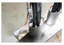
Check the tightness of the screws in the cable glands using hand tools.
