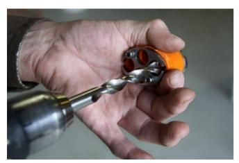
The opening of NAF cable glands. The cable gland is opened with a drill, using the appropriate metallic drill bits. It is important to notice that the size of the drill bit is at least 2 mm smaller than the outer diameter of the cable.
