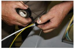
Protect the connector of the grounding wire with insulation tape.
