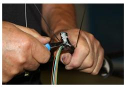
Use a knife to scrape off the white ribbon under the armoring from one of the halves of the cable sheath. Also scrape off the plastic layer on the surface of the armoring.
