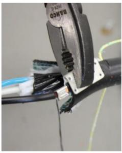
Flatten the end of the cable sheath with pliers and squeeze the connector of the grounding wire onto that half of the sheath.
