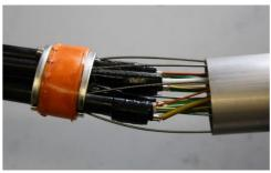
Guide the cables with fibers, steel wires and grounding wires as a bundle inside the joint closure.
