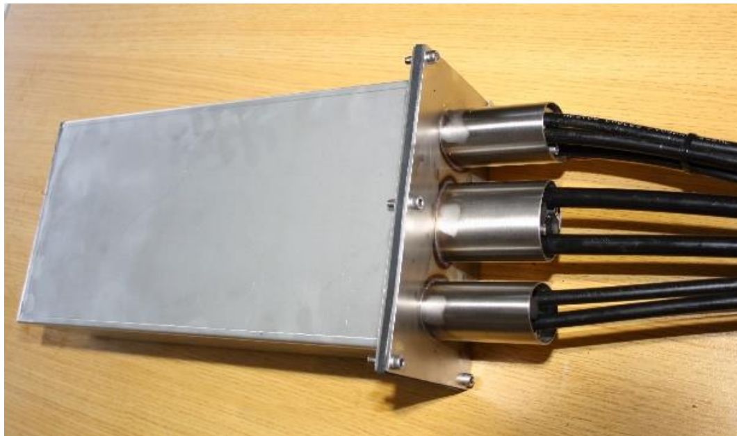
Joint closure installed
