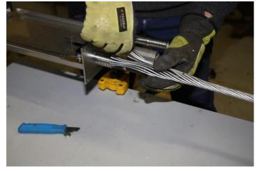
Try to get the wires as evenly as possible over the cable pass-through.
