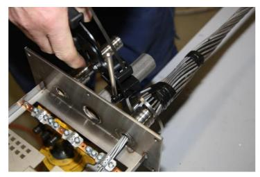
Tighten and cut the wires, preferably with a tool meant for this purpose, as this tool allows the wires to be tightened properly and cut neatly from the root of the steel locking piece.
