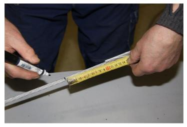
Mark the OPGW wires on the inner layer with their cut-off points at 10 cm from the ends of the outer wire layer.
