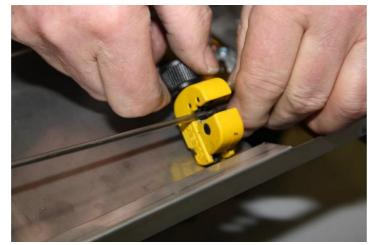
Carefully cut the steel fiber tubes with a pipe cutting tool.
