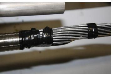
Protect the steel cable ties with insulation tape so that their ends do not penetrate through the shrink that is installed on top.
