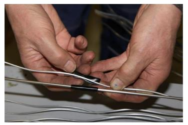
At the same point, rotate the vulcanizing tape around all the wires of the layer.
