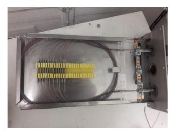
Splice and place the splice protector sleeves onto the splice holders, do it group by group.
