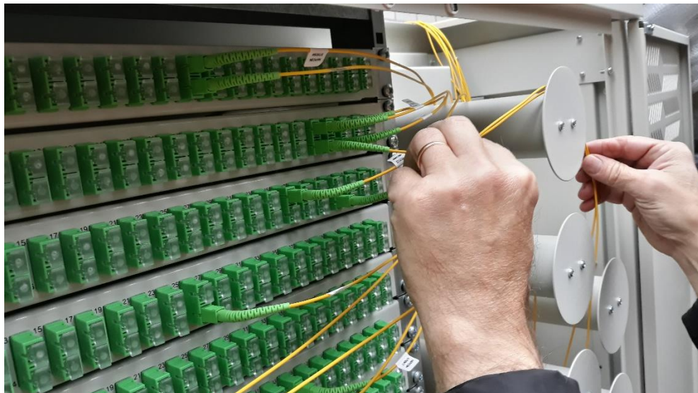
Preinstalled 19" panels with tail cables installed in a cross-connection cabinet.
