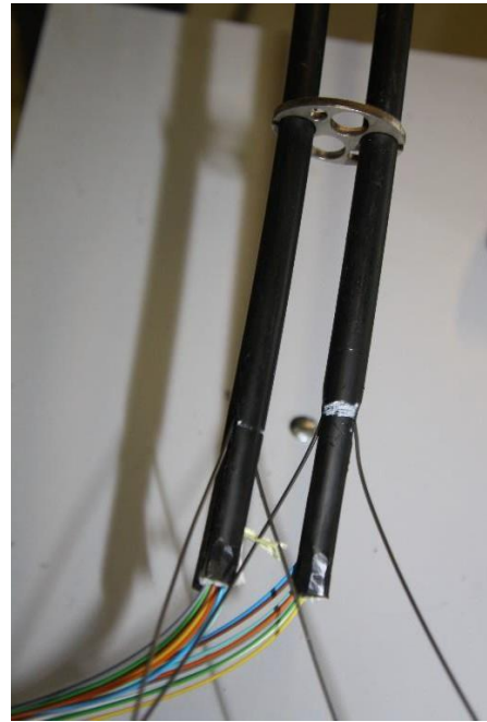
Cable ends pulled through the outer pass-through piece.
