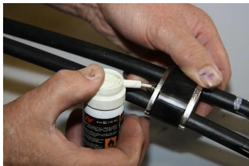
Grease the tightening screws on the cable gland before tightening them.
