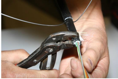
Flatten the ends of the cable with pliers.
