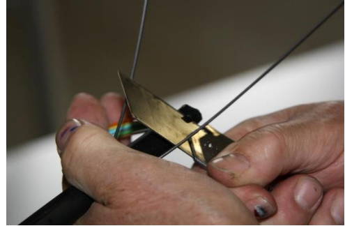
Thin the ends of the cable a little. Thus, they go more easily through the cable glands, but this is also necessary for the installation of earthing connectors.
