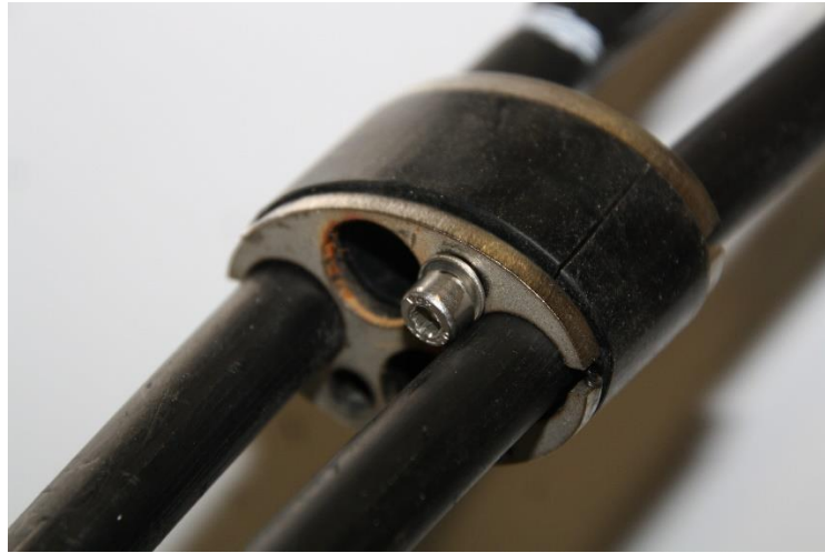
Mechanical cable gland installed.
