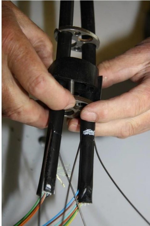
Place the rubber part in place.
