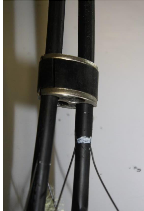
Pull the parts of the whole cable gland together.
