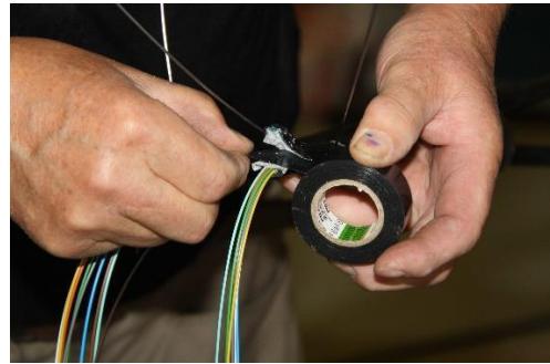
Turn the Flex tubes against the other sheath half and protect them at the end of the sheath with insulation tape.
